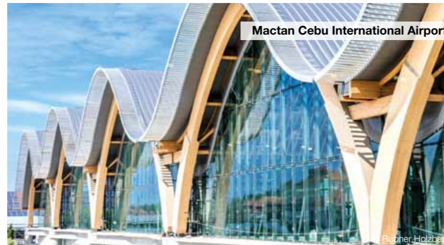
Erstes Flughafenterminal Asiens komplett in Holzbauweise. Asias first airport terminal made entirely of wood.
